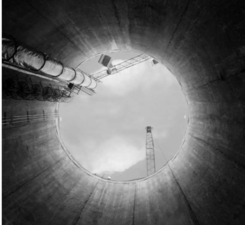
Fig. 5 Diaphragm wall of the L10
